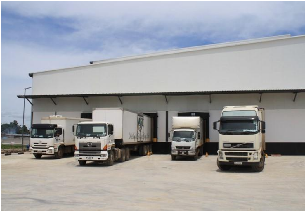
Main Warehouse Receiving Bay Front End
