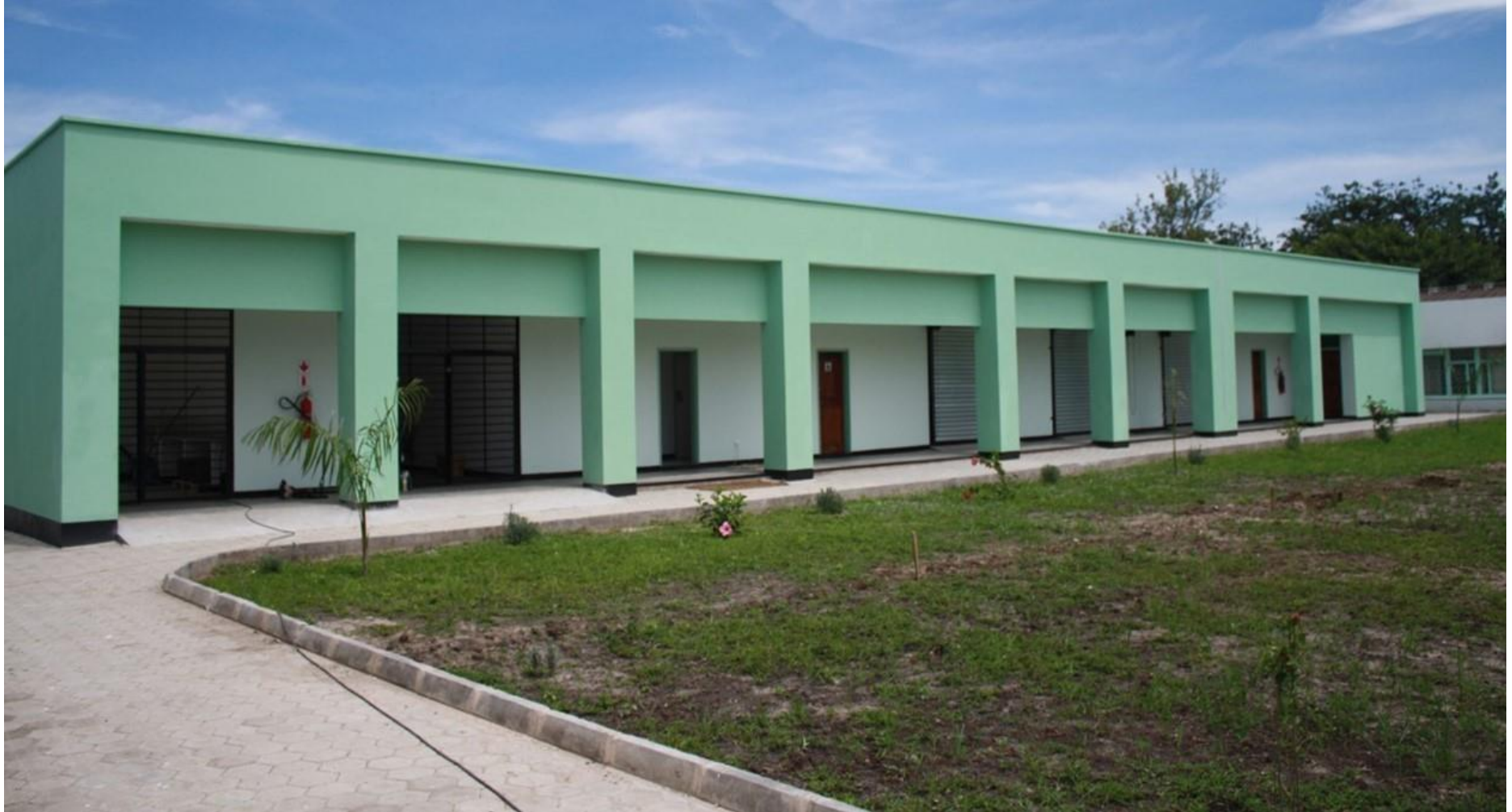
Maintenance Building – Side/Front View
